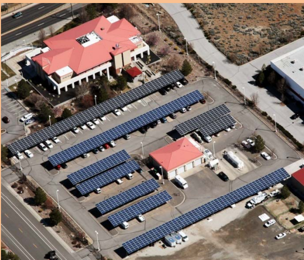
Aerial view of Sparks Police Department Photovoltaic project
